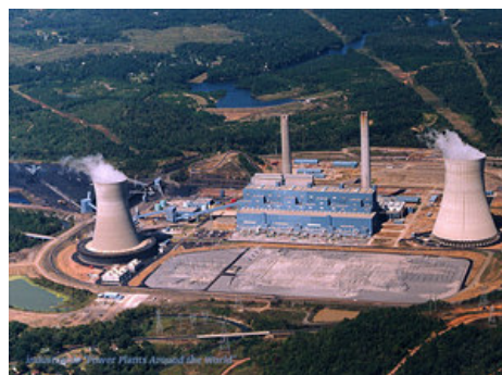
The coal-fired James H. Miller power plant operated by Alabama Power (Photo courtesy Alabama Power)
