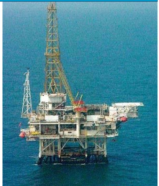
Oil Platform off California's Central Coast
